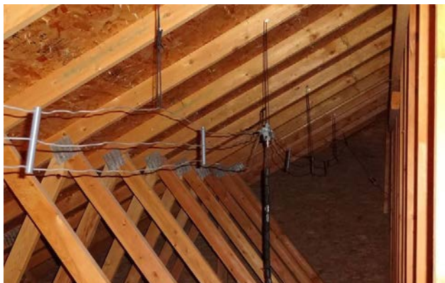
An attic multi-band dipole
